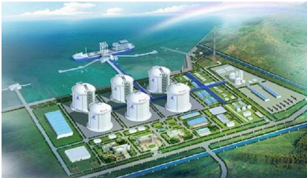
Figure 5: Maheshkhali LNG Terminal
